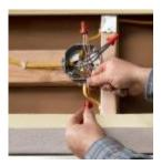
Connect the white wires from the new cables to the white wire from the old cable, and connect the black wires from the new cables to the black wire from the old cable. Connect the ground wires. Cover all open boxes, and then replace the drywall, leaving openings for the fixture and the old box. (Cover the old box with a solid junction box cover plate.)
